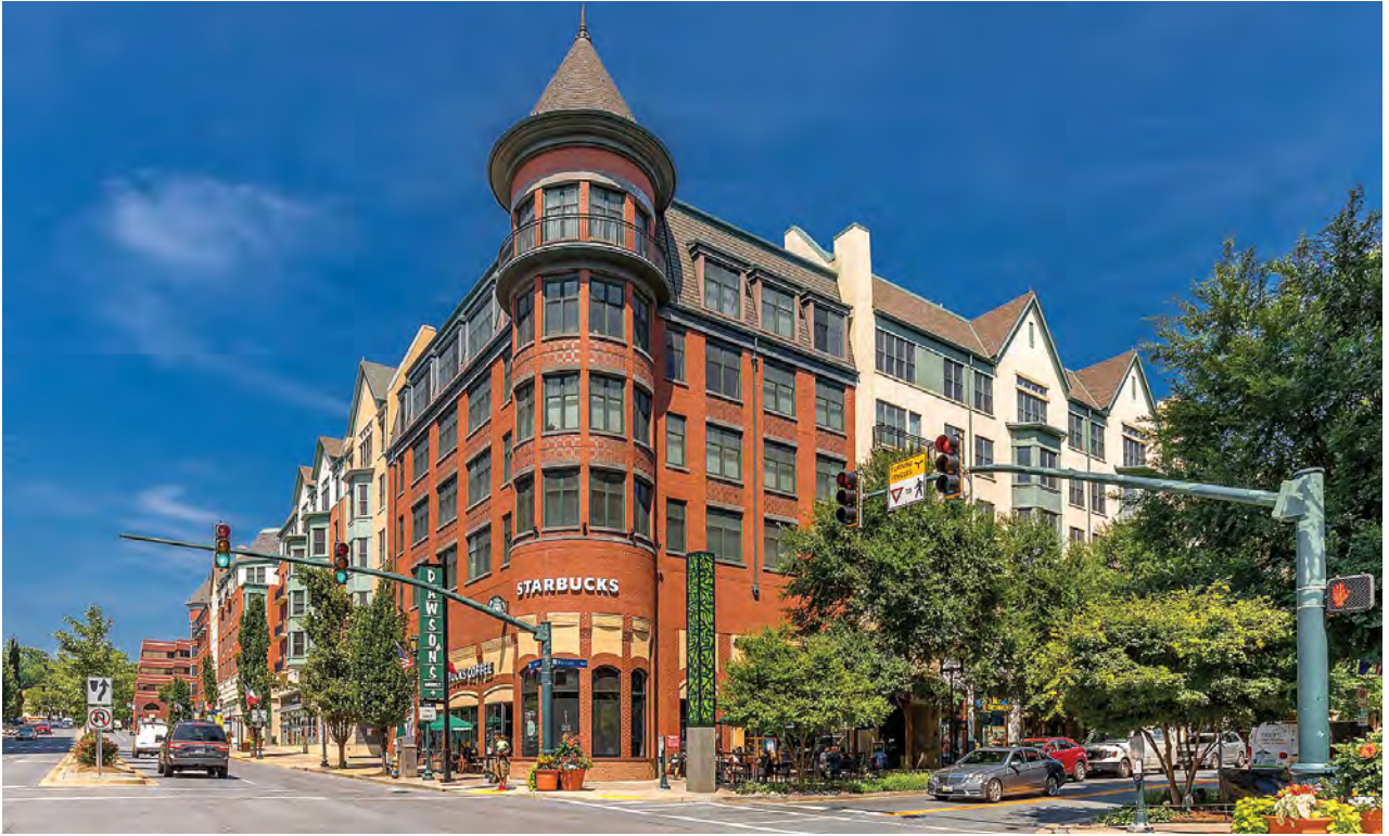
THE FENESTRA AT ROCKVILLE TOWN SQUARE, ROCKVILLE, MD
