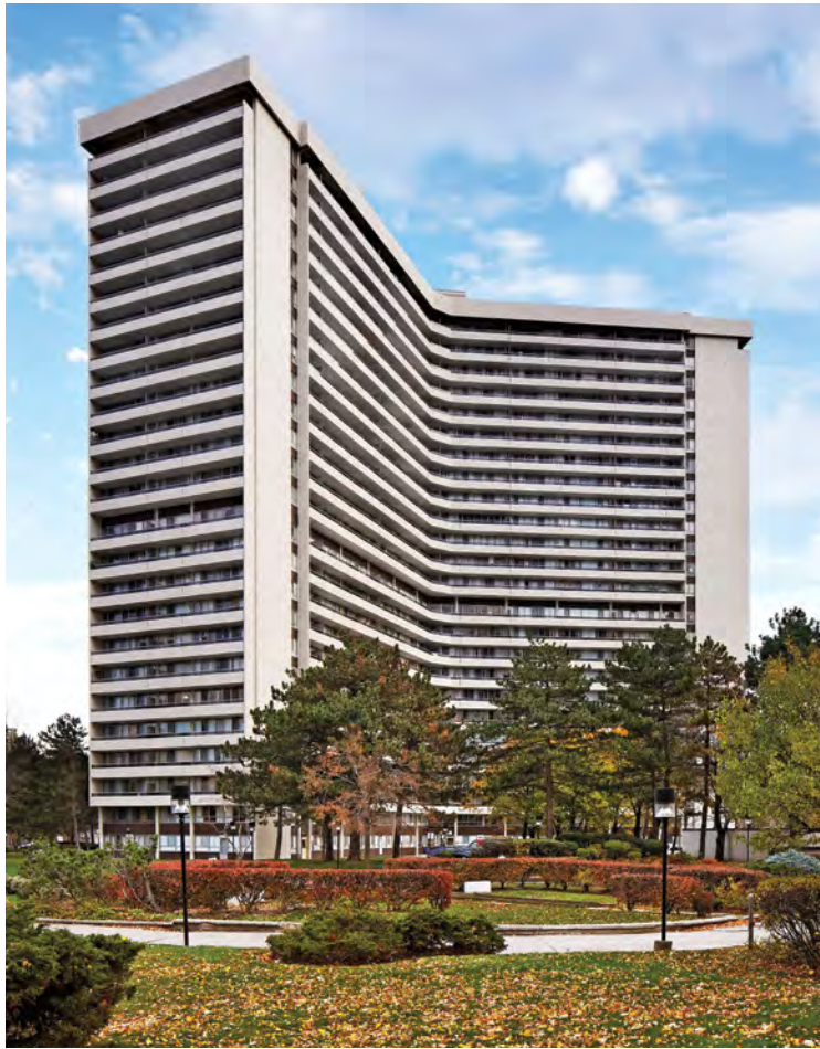
RIDEAU TOWERS III, TORONTO, ON
